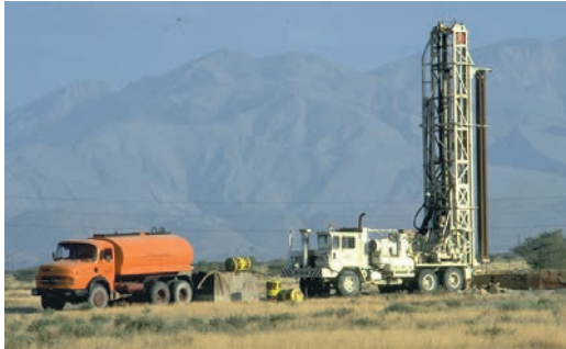
Photograph 5. Drilling for centre pivot irrigation to produce fodder crops on the Batinah coast, Oman.
